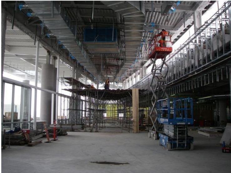
CSB HVAC, Curtain Wall & Ceiling Installation
